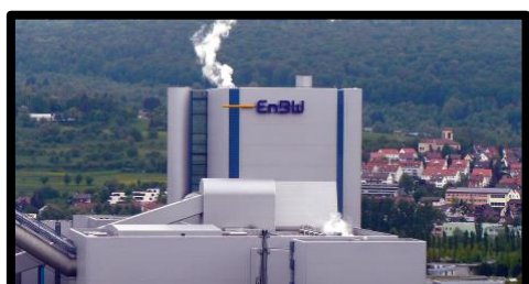
Altbach-Deizisau Power Station Photo: Dierk Schaefer, Flickr
